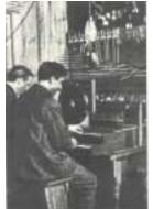
The Telharmonium, also called the Dynamophone, could be considered the world's first "synthesizer". Invented in 1906 by American Thaddeus Cahill, the Telharmonium was an electrical music instrument using rotating electromagnetic generators hooked up to telephone receivers to generate sound. The same principles would later be improved upon to make the Hammond Organ.
