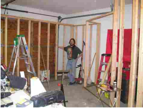
Framing: The first step of construction
