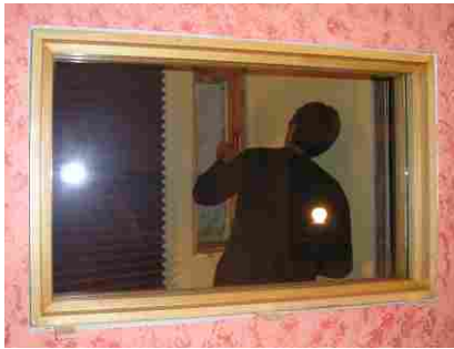
Installing the windows for the isolation booth
