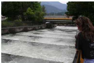
The "Fish Ladder" allows fish to traverse the Bonneville Dam on their way upstream to hatcheries and spawning grounds.
